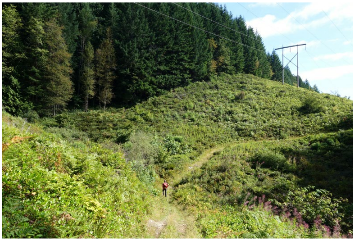
FIGURE 4.1 View eastward along the BC Hydro ROW, near a tributary to Chaster Creek at an elevation of 295 m. Photo DSC09916, August 27, 2020.
