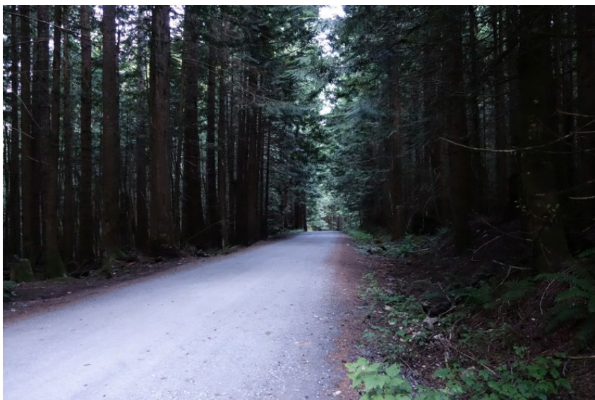
FIGURE 6.8 View of the Sechelt Roberts FSR (7575 Br 3) within the Molyneux Creek watershed at an elevation of 545 m. This example shows a stable road surface with low erosion potential. Photo DSC00079, August 27, 2020.
